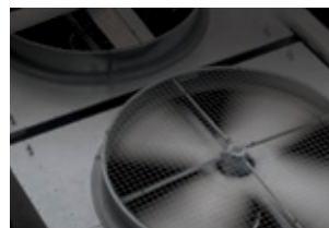
Heating and ventilation
